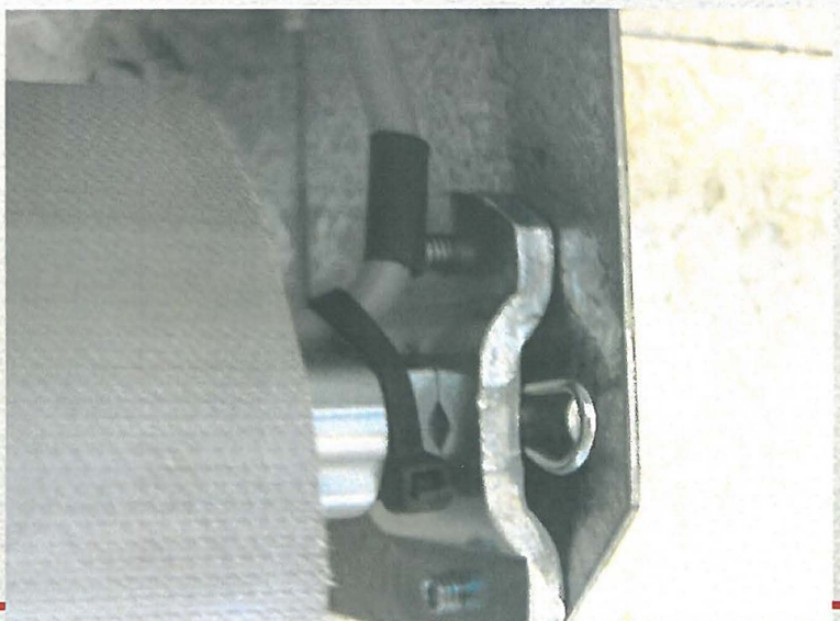
Cable neatly held in place with a cable tie.
